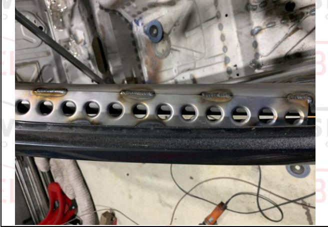
PHOTO 7 FRONT ROLLBAR TO "A" PILLAR ATTACHMENT
